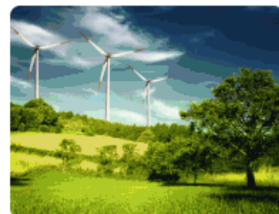
wind power generation
